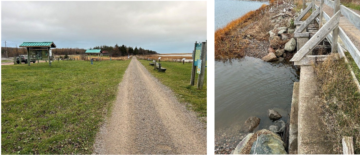
Figure 11: Celtic Shores Coastal Trail showing high water mark (debris line) encroaching on trail surface.
