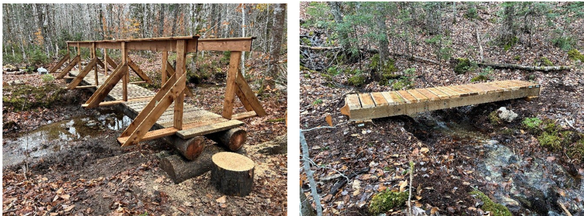
Figure 7: Pedestrian bridge and puncheon spanning watercourses on Little Falls Trail.
