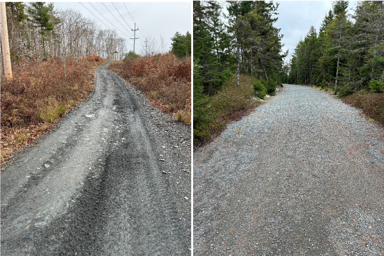
Figure 8: Motorized trails contrasting a graded and crowned travel surface (right) with a rutted and moderately eroded surface (left).
