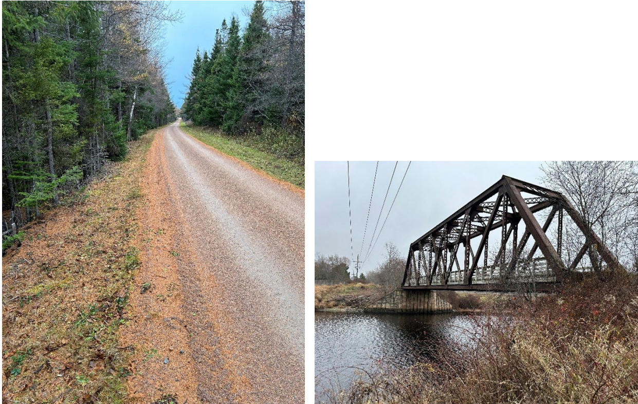
Figure 4: “Rails-to Trails” feature stable trail beds and robust infrastructure.
